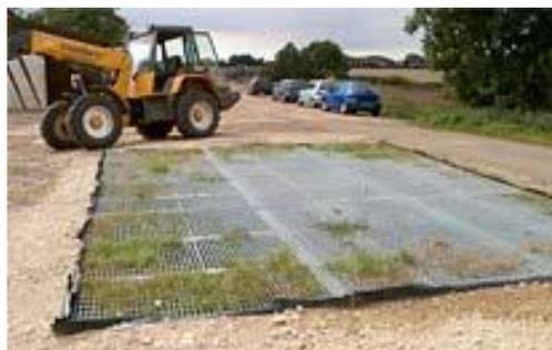
Biobeds can be designed to be either: a) offset – where a separate bunded concrete area is used for sprayer filling and any liquid is drip-fed onto an adjacent biobed: or b) direct – whereby a mesh grid covers the biobed, which can be driven over and any liquid then falls directly onto the biobed below.
